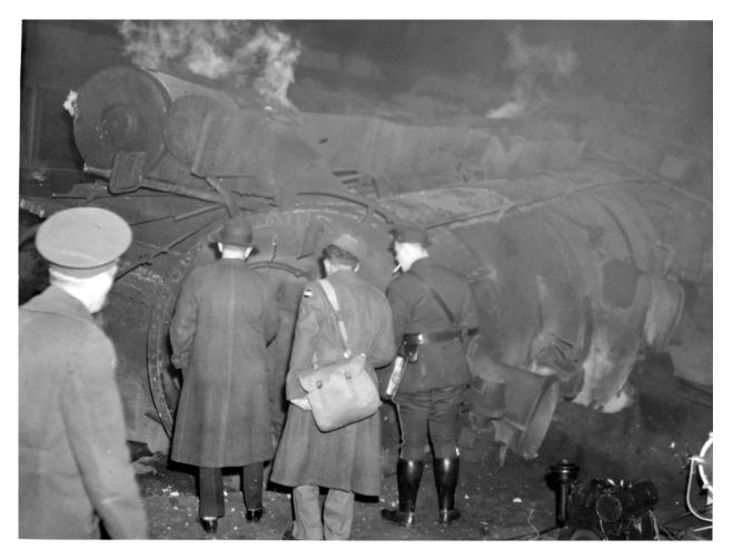
The locomotive of the St. Louisan still has steam escaping when this photo was taken. The passenger train struck a car which lodged under the front four-wheel pony truck. When the locomotive tried to pass over the T&OC crossing at the East Columbus tower it came off the tracks. Photo from the Alex Campbell Collection.
